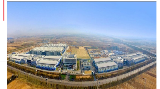
Datong Area | Beijing-Tianjin-Hebei Region 5 Hyperscale Data Center
