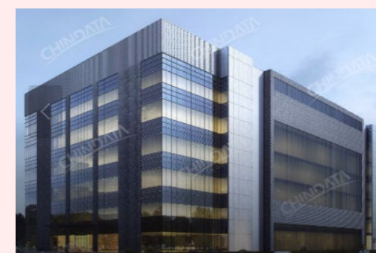
BBY01 Location: Mumbai IT capacity under construction: 20MW
