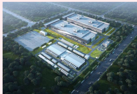
MY06-1,2 Location: Johor IT capacity under construction: 60MW
