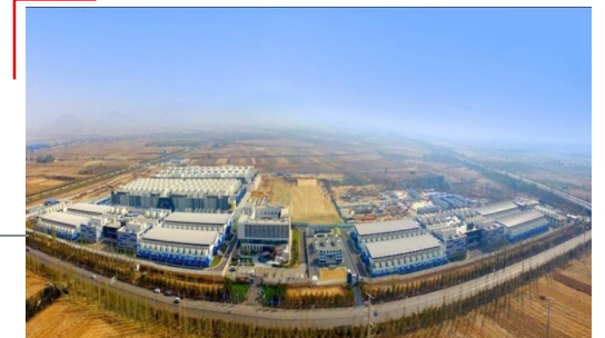
Datong Area | Beijing-Tianjin-Hebei Region 6 Hyperscale Data Center
