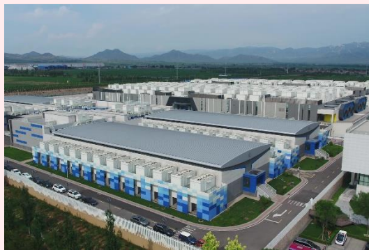
CN01 Location: Greater Beijing Area IT capacity in service: 36MW
