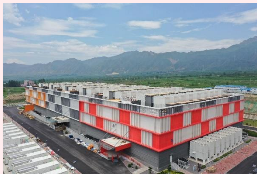
CN07 Location: Greater Beijing Area IT capacity in service: 29MW
