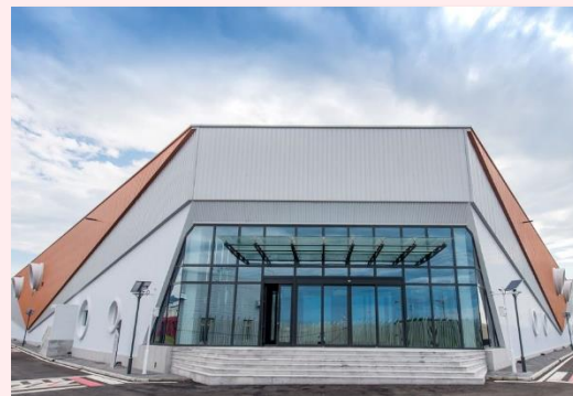
CN05 Location: Greater Beijing Area IT capacity in service: 23MW
