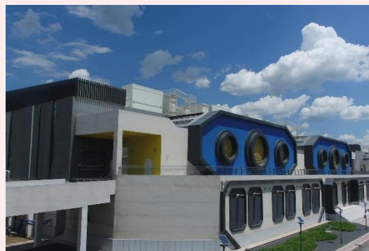
CN08 Location: Greater Beijing Area IT capacity in service : 51MW
