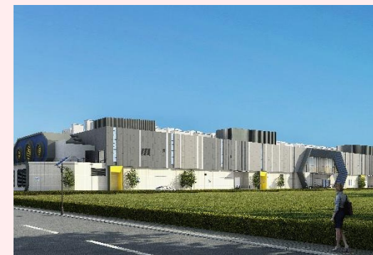
CN15 Location: Greater Beijing Area IT capacity in service: 52MW
