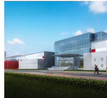
CN03 Location: Greater Beijing Area IT capacity in service: 17MW
