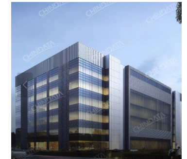
BBY01 Location: Mumbai IT capacity under construction: 20MW
