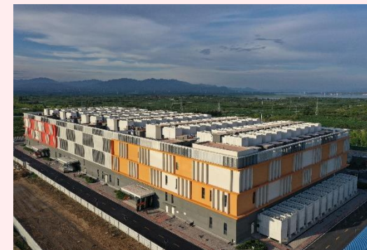
CN06 Location: Greater Beijing Area IT capacity in service: 30MW
