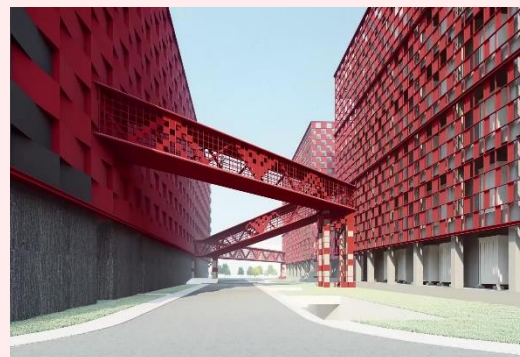
CN11 Location: Greater Beijing Area IT capacity in service: 119MW
