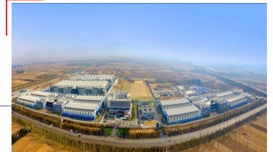
Datong Area | Beijing-Tianjin-Hebei Region 5 Hyperscale Data Center
