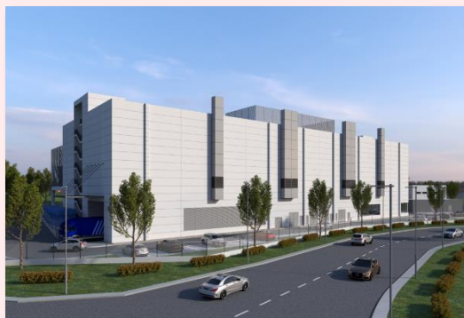
MY03 Location: Cyberjaya IT capacity under construction: 16MW
