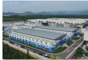
CN01 Location: Greater Beijing Area IT capacity in service: 36MW
