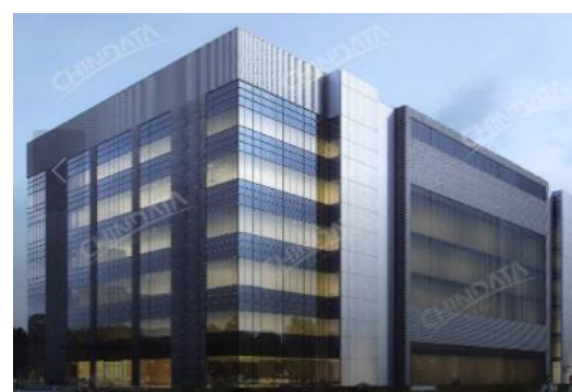
BBY01 Location: Navi Mumbai, India IT capacity in service: 20MW
