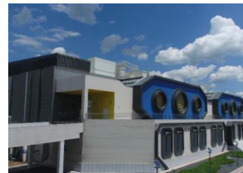
CN08 Location: Greater Beijing Area IT capacity in service : 51MW
