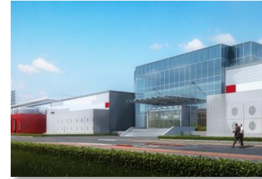
CN03 Location: Greater Beijing Area IT capacity in service: 17MW
