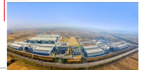
Shanxi Datong Area | Beijing – Tianjing – Hebei Region | 8 Hyperscale Data Centers
