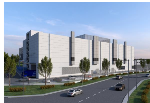
MY03 Location: Bukit Jalil, Malaysia IT capacity in service: 16MW
