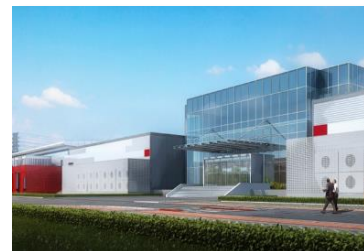
CN03 Location: Greater Beijing Area IT capacity in service: 17MW
