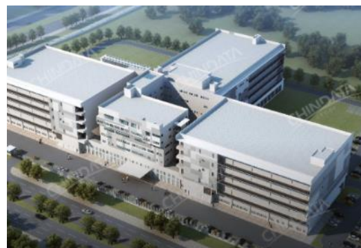
MY0102 Location: Cyberjaya, Malaysia IT capacity in service: 20MW
