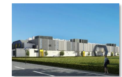
CN15 Location: Greater Beijing Area IT capacity in service: 52MW
