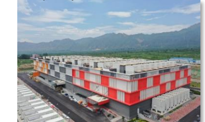
CN07 Location: Greater Beijing Area IT capacity in service: 29MW
