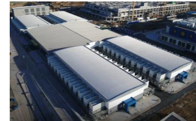
CN14 Location: Greater Beijing Area IT capacity in service: 18MW
