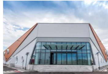
CN05 Location: Greater Beijing Area IT capacity in service: 23MW
